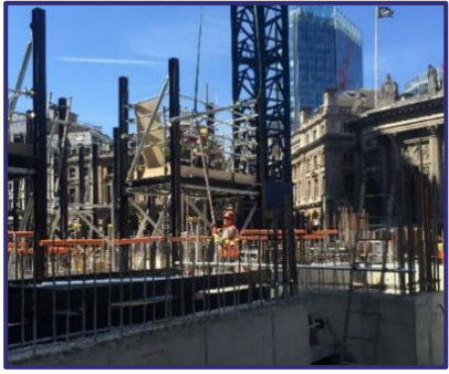
Rigs on the top of the two core walls
