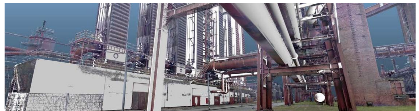
Point cloud with an overlaid CAD model, Zeche-Zollverein, Essen, Germany
