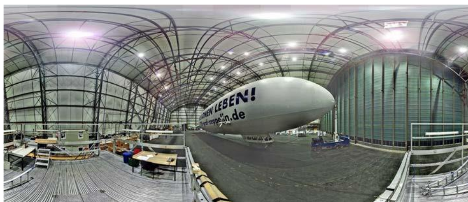
Scan of the Zeppelin NT-Hangar
