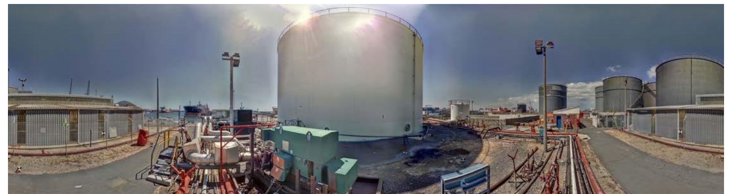
Point cloud of a site with strong backlight. Source: Satmap Solutions/HORTS Solutions, South Africa
